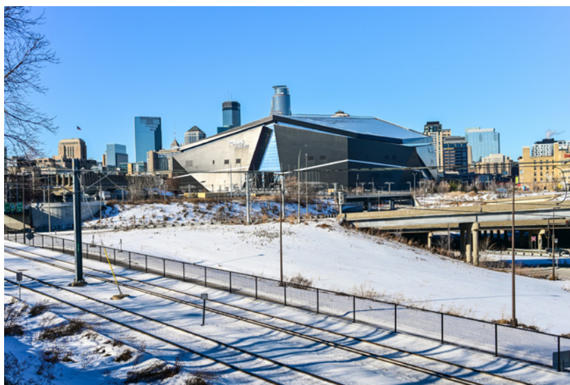
Minnesota Vikings US Bank Stadium Minneapolis, Minnesota (Usa).
